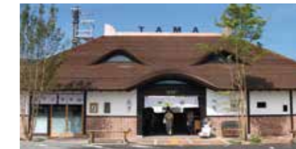
The roof of Kishi Station is made using a traditional Japanese cypress bark-thatched style in the shape of a cat's face.
